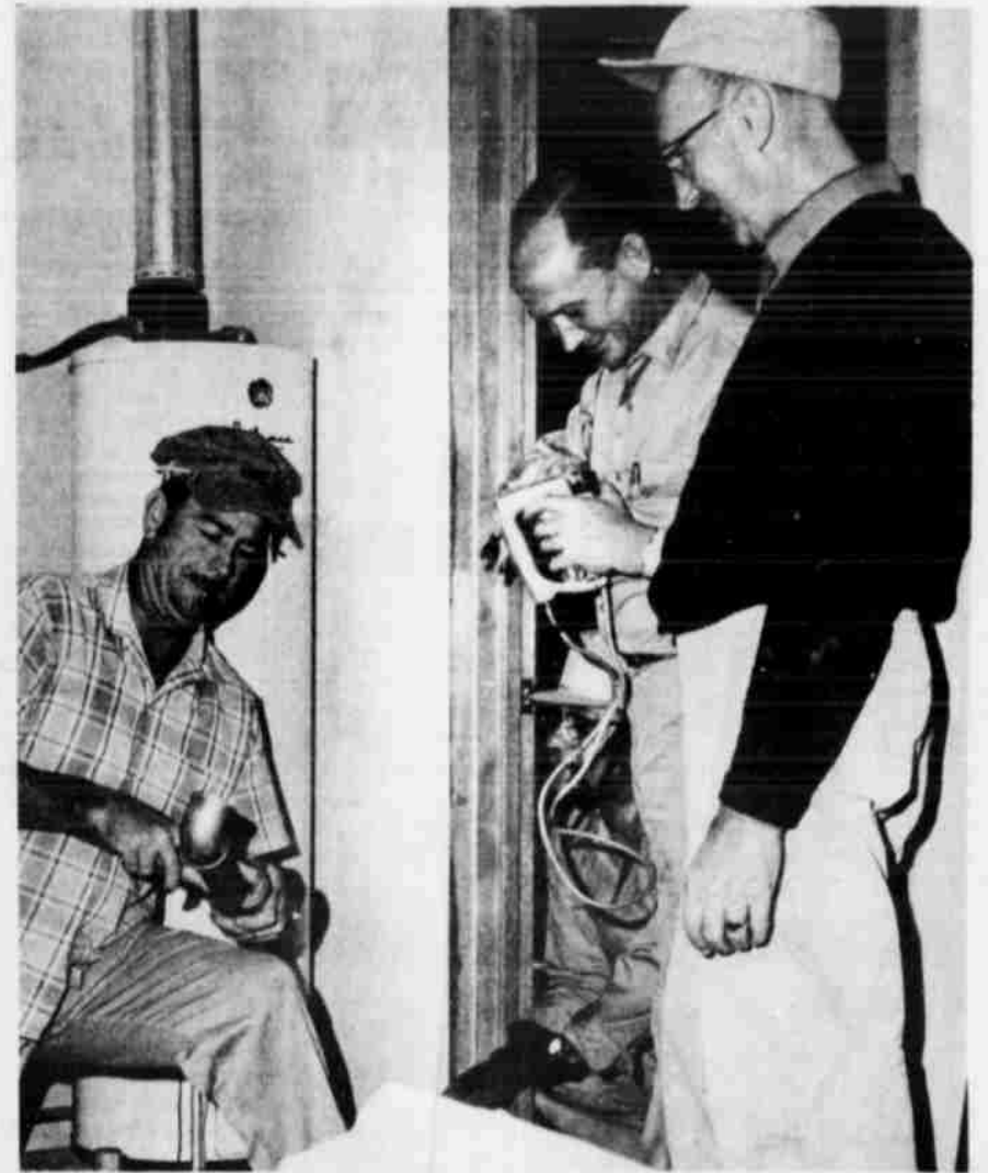
FOUR LITTLEFIELD preachers are busy this week knocking out partitions, putting in plumbing and getting the Antioch Baptist Church ready for its new role as headquarters for the Satellite School that is beginning its third year here. Rev. Clem Sorley, Rev. Doug Morton, and Rev. Louis Wetzel are getting the kitchen ready for occupancy within the next two weeks. Sustaining donations of $100 a month are needed for the school, in addition to tools for a sheltered work shop, kitchen supplies and some good carpets.
