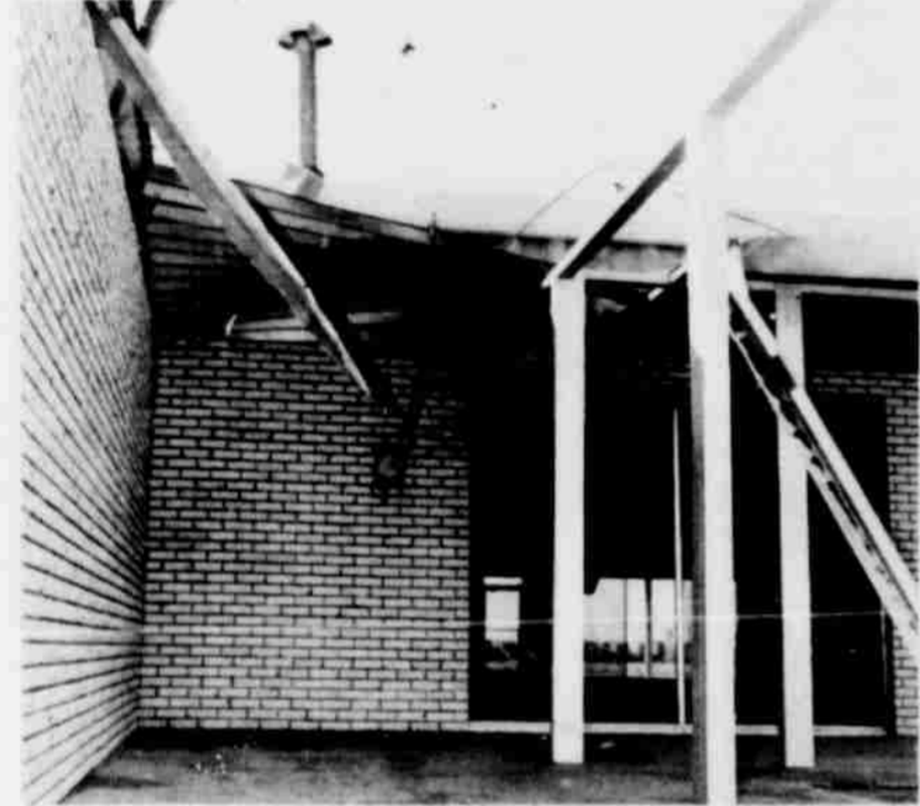
AN AWNING was blown from the north side of the former Rogers Furniture Building and down this west side of the building to the corner of another north wall. Also damaged were two large plate glass windows on the north side. (Staff Photo)
