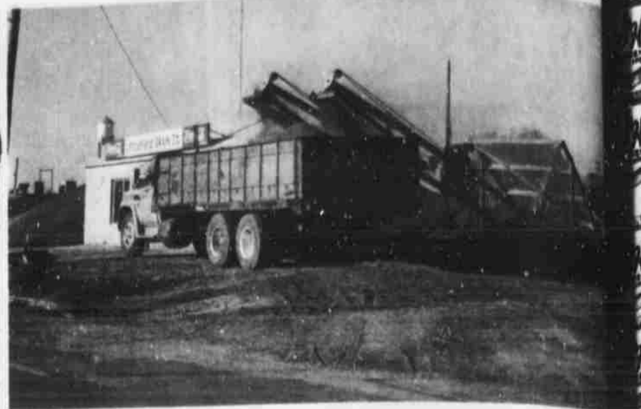
CLEANUP PROCESSES were nearing completion by presstime Wednesday. Littlefield Grain Co. According to Doyle Dean, owner of the elevator which burned 18, approximately two-thirds of the grain will be salvaged. Front loaders picked grain and dumped it through a huge screen. The screened grain was re-screened and it was loaded on trucks.
