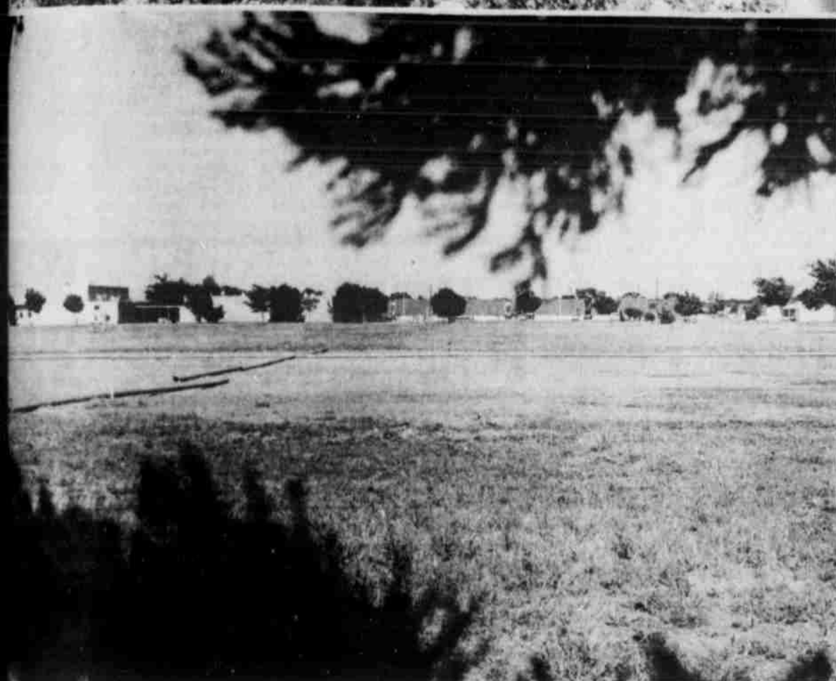
SCHOOL PROJECTS have begun the summer vacation began. The ground is prepared for
