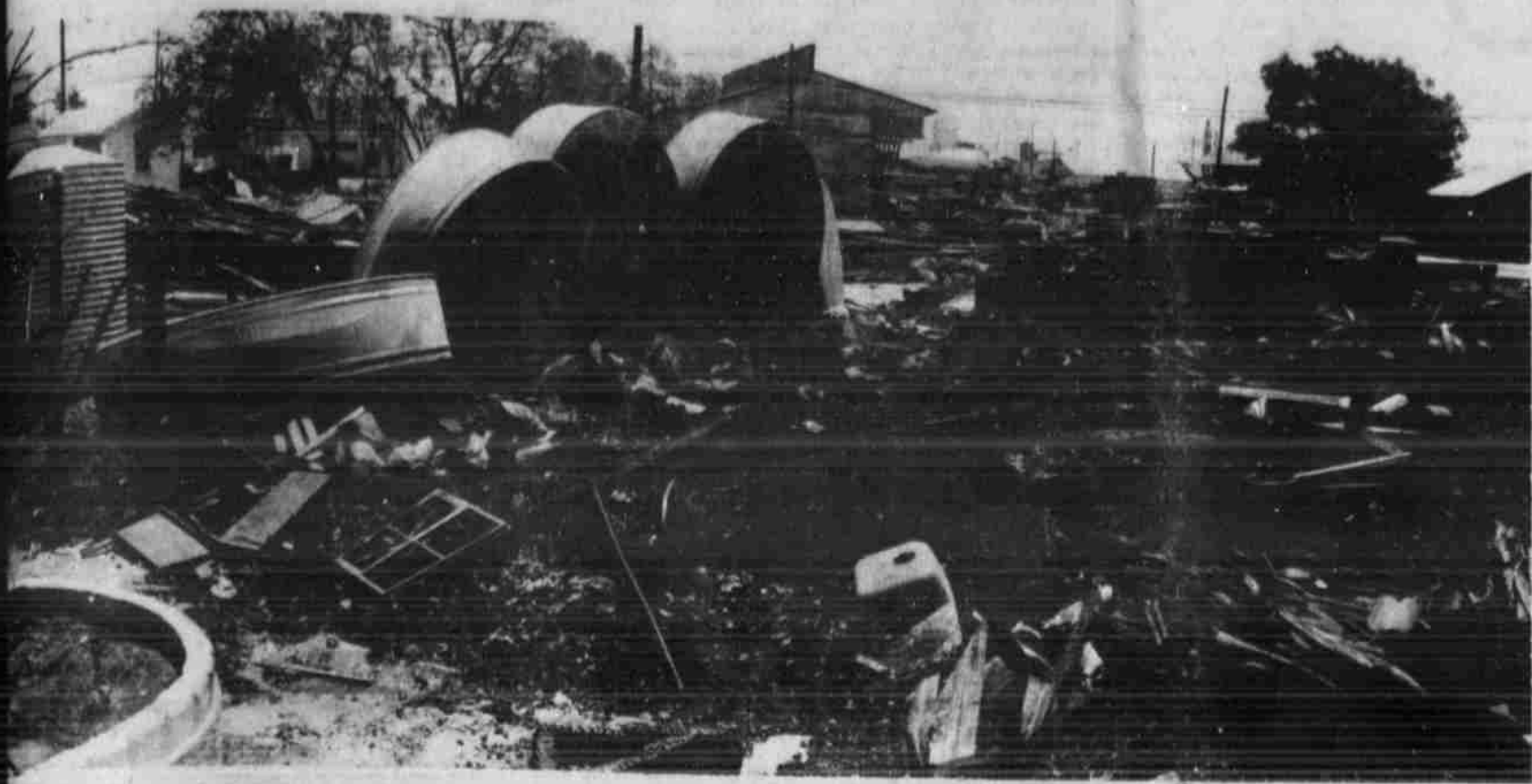
Damages amounted to more than $200,000. Shown here are the charred remains of an evergreen tree in a street planter on Phelps Avenue, (left), various hand tools (lower right), rolls of wire, buckets of paint, water heaters, lumber, stock watering tanks and sheet metal.
