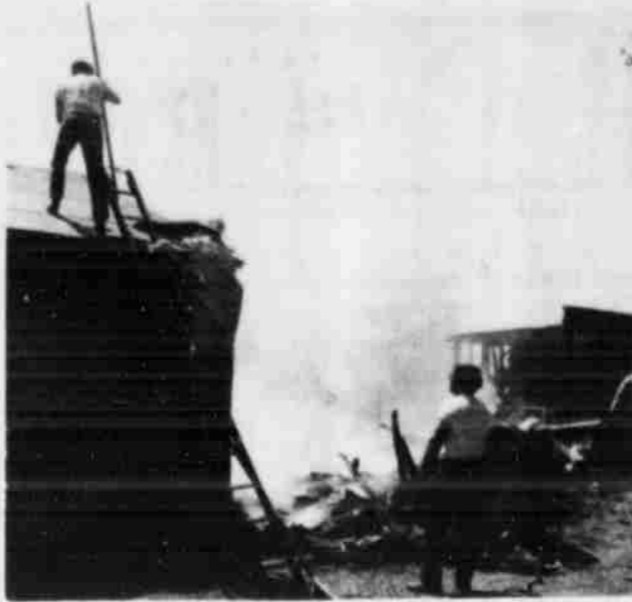
TWO BUILDINGS , owned by Manuel Hernandez and located at 295 N. Wicker, were extensively damaged by fire Tuesday during the wind storm. Firemen work to extinguish a fire on the roof of the front building, which housed the property of Hernandez' mother, who died about three weeks ago.
