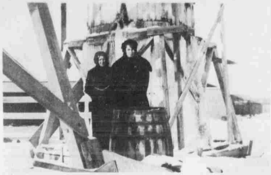
Frozen water tank
