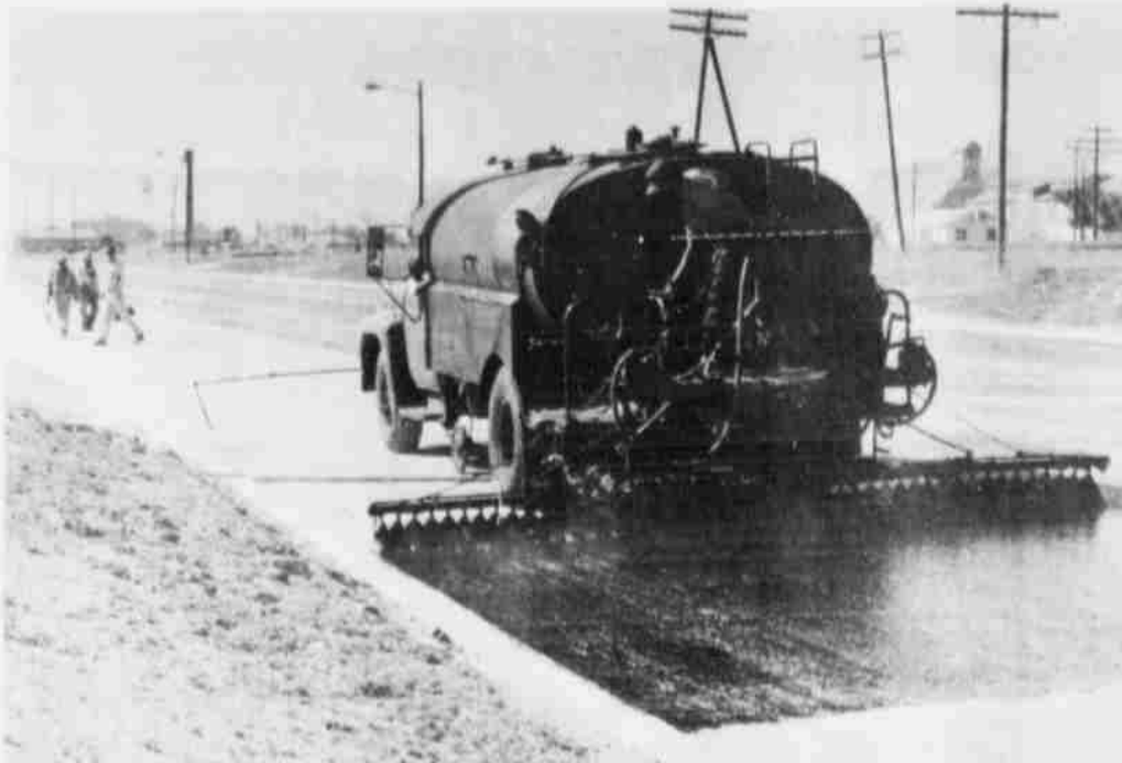
DELANO AVENUE is getting its surface coating this week. The first oil coating has been sprayed on and in the last few days the asphalt and gravel final coat is being added.
