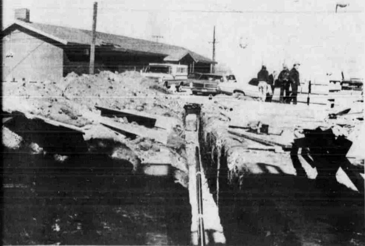
MATIC TUBING for First Bank's proposed new banking facility is being used to conduct business transac-
