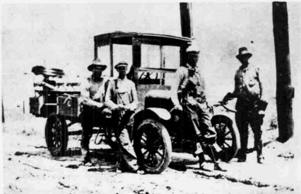
SERVICE TRUCK — These crew members relax a moment after erecting an electric transmission line. This 1920 version of a line construction truck had no automatic lifting equipment on it.
