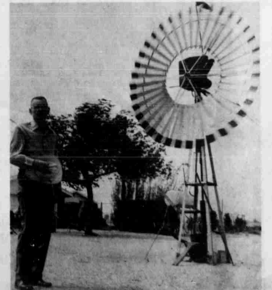
EVEN IN "hang onto your hat" winds, Gus Parish's windmill pumps about 25 strokes per minute. "Poppa" Gus stands by a windmill tower at his home south of Earth. The slow pace of the pump rod in high winds is the result of the vane or tail that acts as a governor. Conventional windmills pump 40 or more strokes per minute in high winds. This churns up sand that wears out windmill parts and causes an uneven flow of water.
