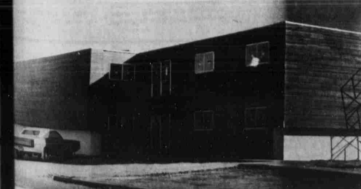
OAK TERRACE APARTMENTS NEARING COMPLETION
