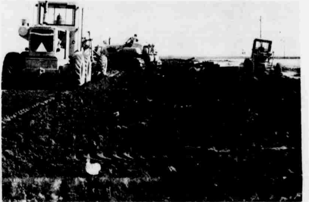
CONSTRUCTION on the overpass at intersection of Highway 84 and FM 54 was begun last week. Various types of road machinery are busy loosening, packing and shifting dirt in the construction area.
