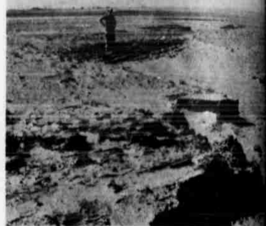
PAT RICE, Soil Conservation Service technician, needed repairs on terraces that were washed out on farm south of Littlefield following a hail storm and heavy spring rains.
