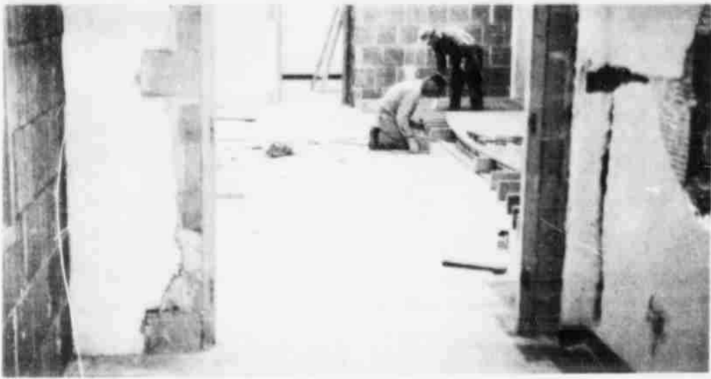
WORKMEN BUSY IN REMODELING
