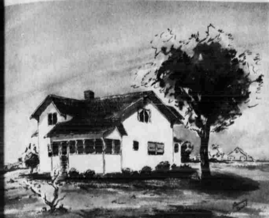
IN 1917, the "Miller House" stands as majestic as ever, unaware of the time. One of the first farm houses built in the Littlefield area, its size of the great expectations early settlers had for the High Plains of Texas. Henry Brandt family moved into the house in 1929, coming here from the Grande Valley, and living in the house until recent years. The house stands the west of Littlefield, and can be seen from the Amherst Highway. (Sketch by Benny Goss.)
