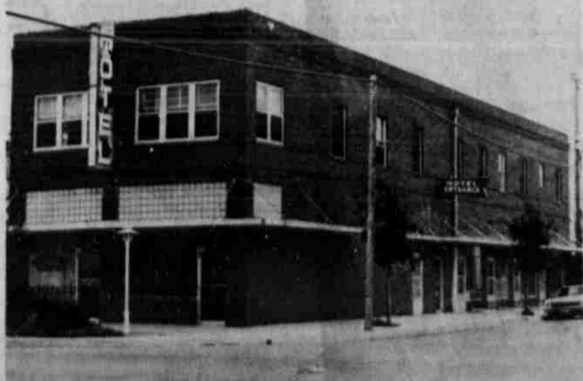
THE RUMBACK HOTEL is being made into five modern apartments and will be opening soon. Upstairs of this building has been serving as a 20-room hotel for approximately 40 years, and is one of the first early-day brick buildings constructed in Littlefield. [Staff Photo]
