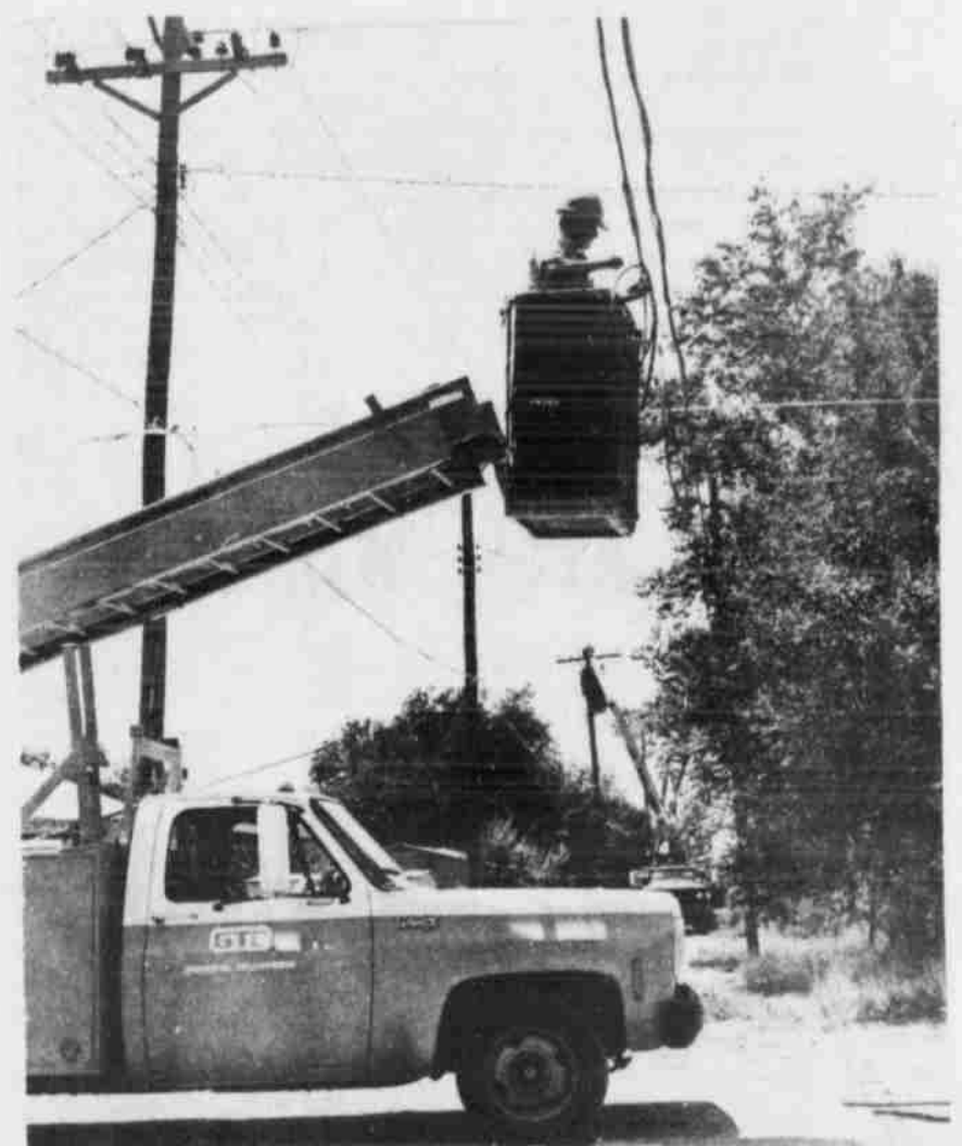
A TELEPHONE CABLE containing 55 pairs of wires to the Anton Exchange were cut in two shortly after noon Tuesday when a truck went down Eastside between East 8th and East 7th, caught the cable, shook the lines, knocked local telephone lines out of service and caused a Southwestern Public Service Co. transformer to burn out. Here, repairmen for both companies are at work. In the foreground the telephone lines are being spliced, while in the background a new transformer is being installed. (Staff Photo)
