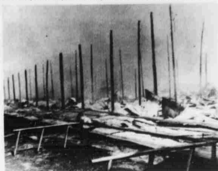
elevator as it burned down from a fire that started in the top of the structure. About three hours later, the empty elevator and storage building were burned to the ground.
