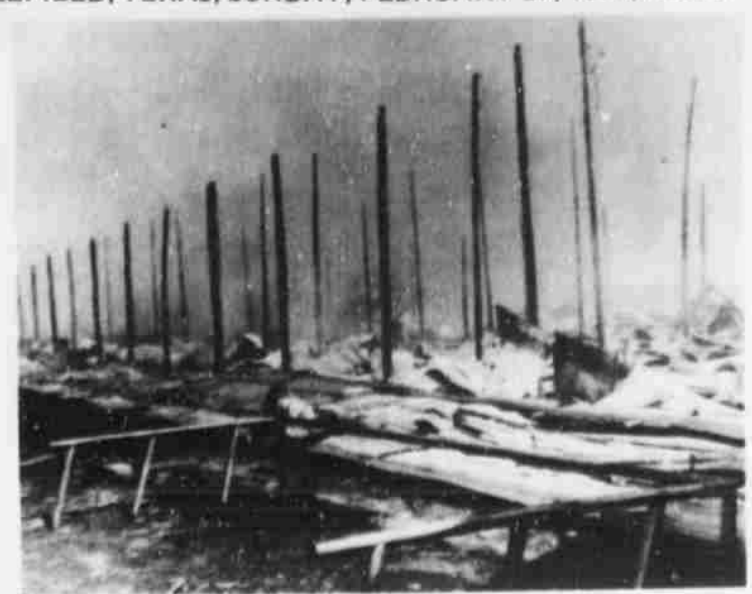
elevator as it burned down from a fire that started in the top of the structure. About three hours later, the empty elevator and storage building were burned to the ground.
