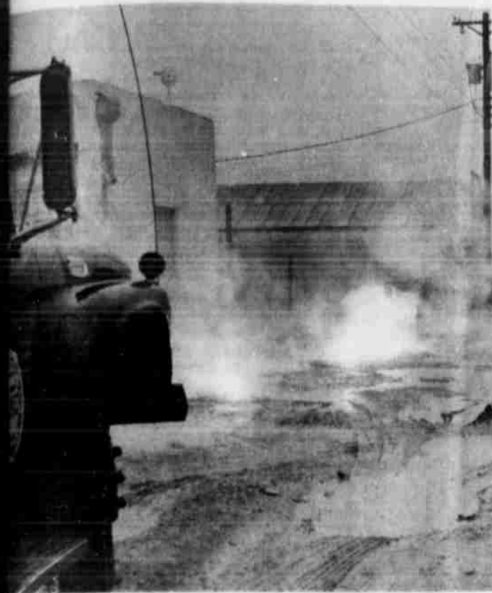
WORKING STRUCK a highline pole behind Littlefield Steam Laundry Saturday morning, and a high-voltage wire lit up the rain-drenched area with an orange-colored hue before servicemen could cut the wire off the flow of electricity.
