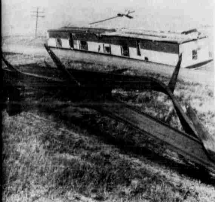
LARGE MOBIL HOME was whipped by high winds shortly after noon and was severed from the wheels and frame while it was being blown by a sand storm that struck Littlefield and the South Plains ahead of a cold front that dropped temperatures to below zero in some places. (Staff Photo)
