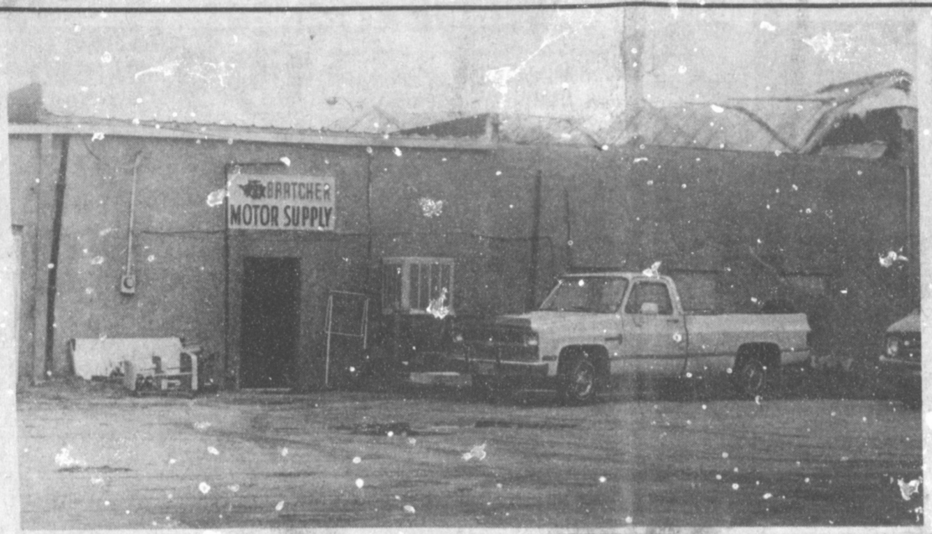
A ROLLED UP ROOF ON THURSDAY -Thursday evening, black clouds moved from north over Muleshoe depositing nearly three-fourths of an inch of rain. However, just at the beginning of the rainstorm, heavy winds drew the cloud into town. One victim of the storm was the roof of Bratcher Motor Supply, which rolled up due to the intense windstorm. No other measurable damage was reported due to the storm. Intermittent rain fell all day on Friday, and as evening approached, black clouds were again rolling in from the north. (Journal Photo)
