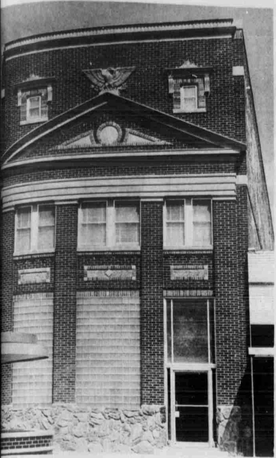
FIRST NATIONAL Bank got a new facade last week. The maroon file on the front moved and replaced with this field stone. (Staff Photo)
