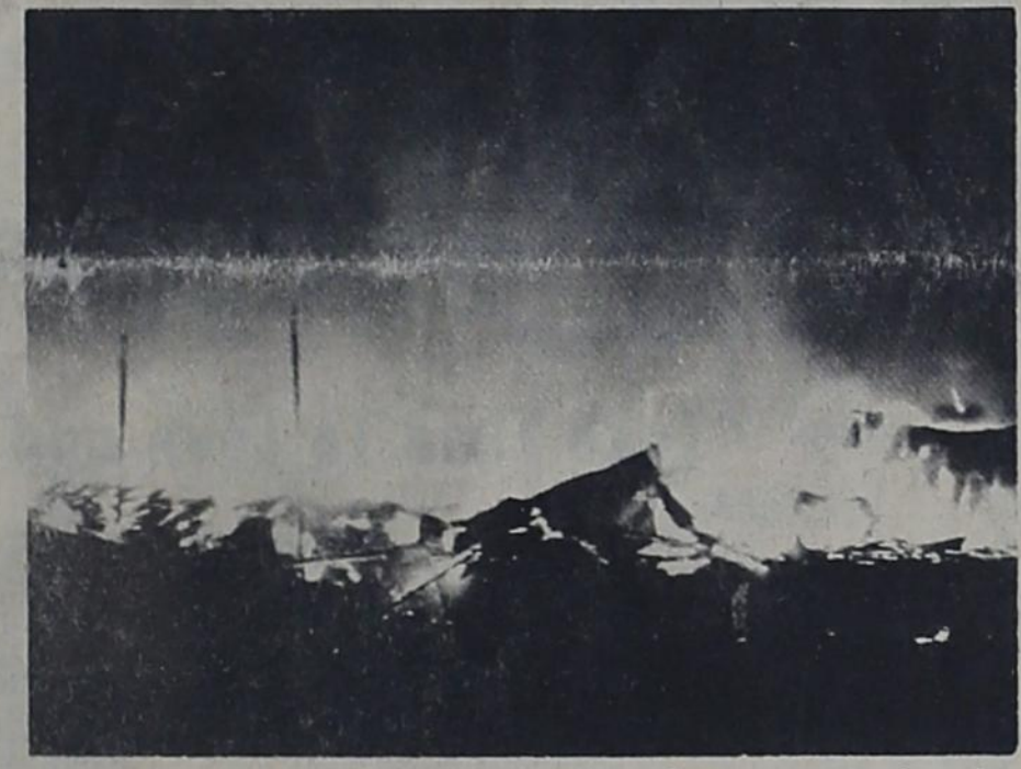
The walls came tumbling down -- When firemen arrived on the scene of the largest fire in Farwell at U.S. Seed Co. in years, shortly after 2 a.m. Wednesday morning, it was too late to save this structure. All firemen could do was to stop the fire from spreading to nearby buildings.
