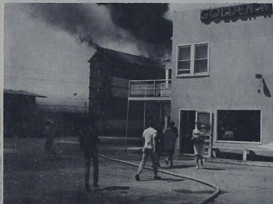
Employees evacuate the office building as the fire increased in intensity.
