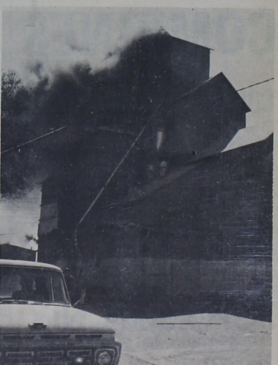
Smoke almost completely enveloped the building as it began pouring forth following a dust explosion inside the elevator.
