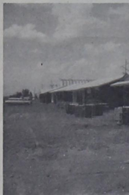
The four houses on Eighth Street being constructed by Bill Nance, building contractor, are nearing completion and should be ready for occupancy by middle of the summer. They are three and four bedroom houses of brick veneer, and may be bought by securing loans through Farmers Home Administration office in Farwell.
