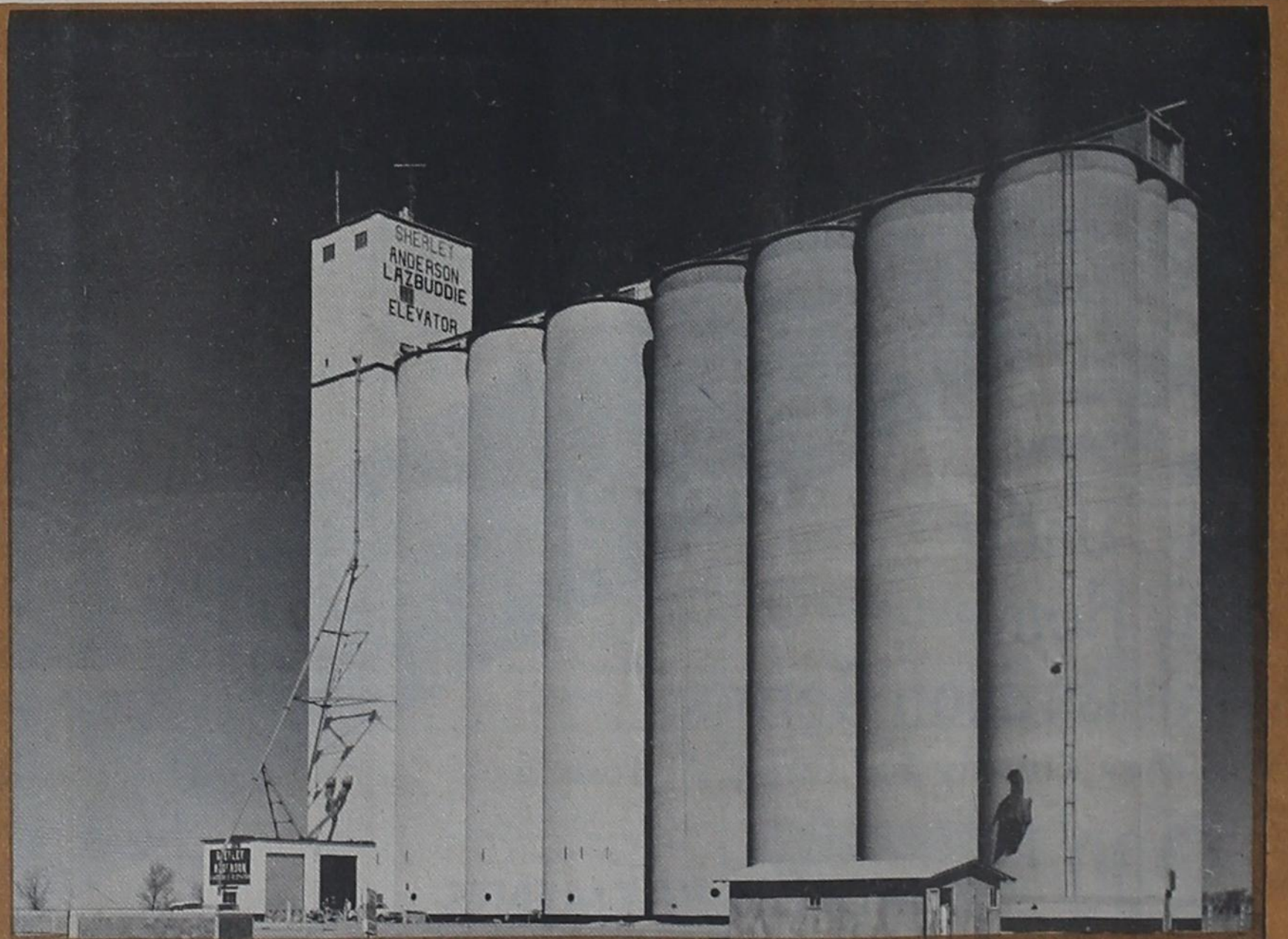
Sherley - Anderson LAZBUDDIE ELEVATOR
