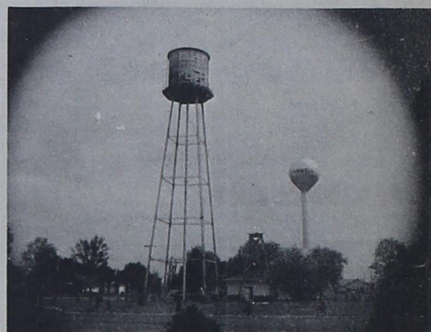
THE OLD AND THE NEW -- as man progresses, so do his means of storing the precious fluid he has removed from the earth.
