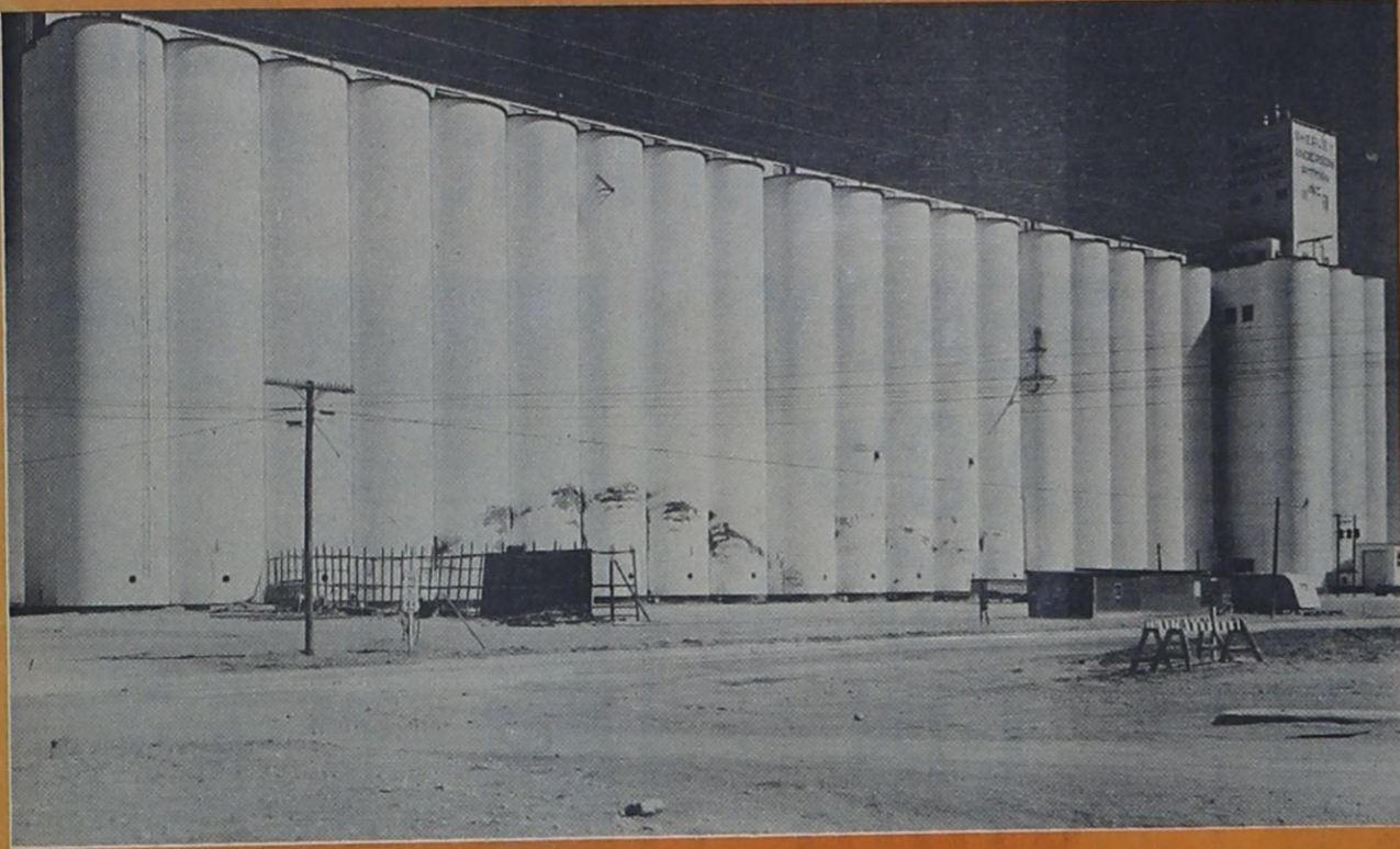
SHERLEY-ANDERSON-PITMAN, INC. - FARWELL JOHNIE WILLIAMS--FRED CHANDLER--SUSIE HAMMONDS
