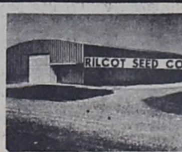
NEW WAREHOUSE - LUBBOCK HIGHWAY - LITTLEFIELD BUSTER OWENS
