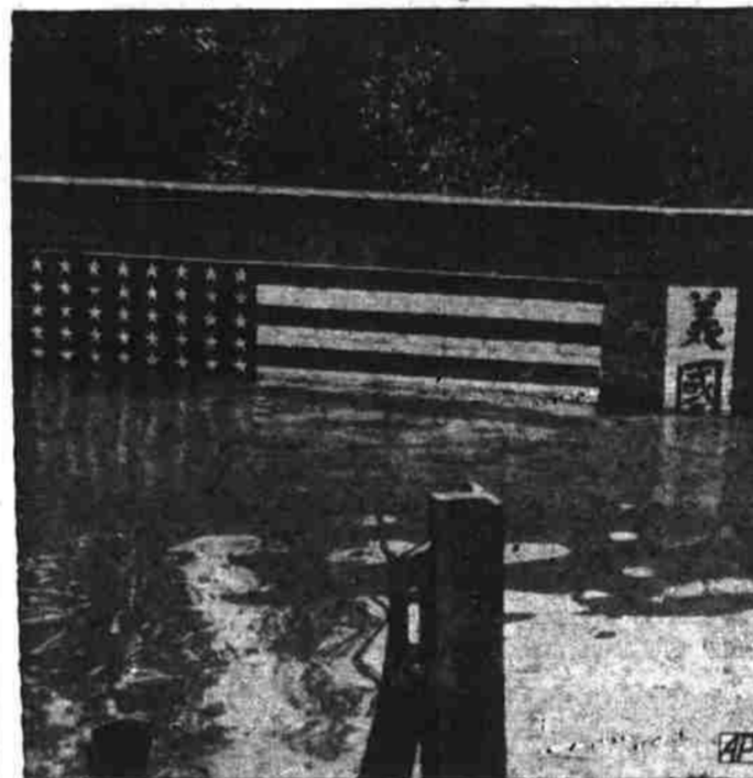
BATH FOR 'OLD GLORY' —When floods from the Hai river inundated Tientsin, China, causing damage estimated at $108,000,000, this flag on an outside wall of the American Marines club got a good wetting. Water's six feet deep here.
