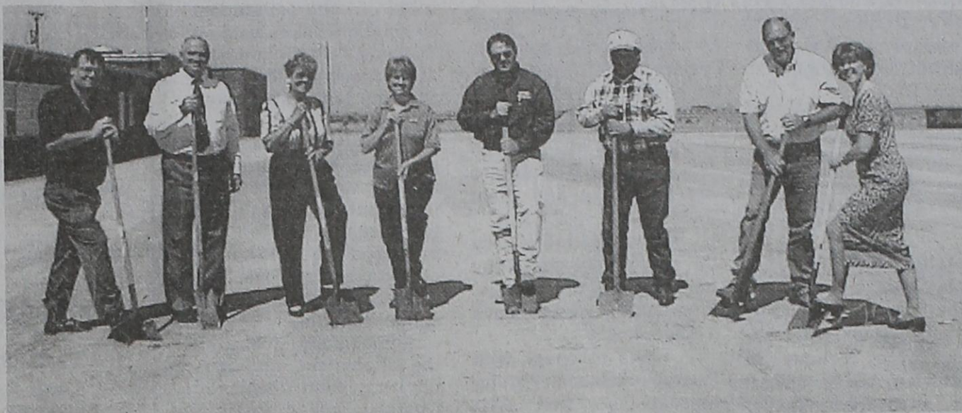
The groundbreaking for the new Texico High School gymnasium was held on Aug. 3. Among the dignitaries present for this very special event were, from left, Scott Barthel, representing the State Board of Education; Texico High School Principal David Hutton; state Rep. Anna Crook, whose district includes the northern half of the Texico School District; Texico school board members Deborah Autrey, Richard Hadley, Ted Richardson and Randy Cain; and state Sen. Shirley Bailey, of Hobbs, whose district includes Texico Schools.
