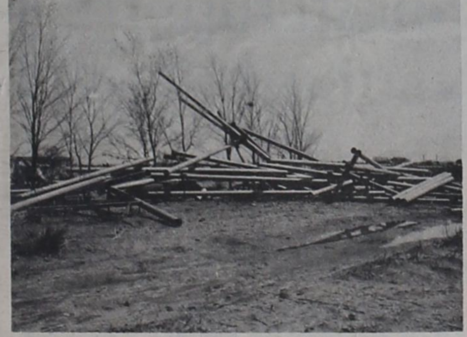
PICK-UP STICKS ANYONE? -- These lengths of aluminum pipe which were stacked neatly in rows at the Clyde McDaniel farm south of Texico were twisted and turned by Thursday's winds to resemble a pile of pick-up sticks. Other damage included uprooting of many trees in the area along with scattered debris.
