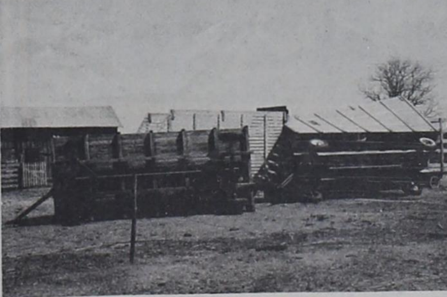
TOPSY-TURVY TRAILERS -- Thursday night's storm played topsy-turvy with these cotton trailers at the T. J. Kittrell farm southwest of Texico. An apparent twister or tornado hit on the farm, destroying a tool shed and unroofing a hog shed. Two cotton trailers were overturned and the trailer which is upright in the background was standing end to end with the trailer in the right of the picture and was apparently sucked up and put down facing the opposite direction without ever being turned over.
