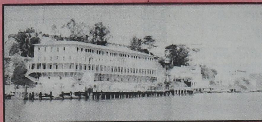
The dock in front of the prison is an inviting white structure.
