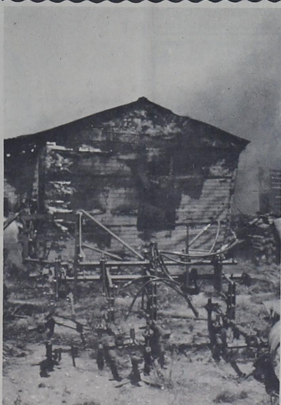
BLAZE CONSUMES HOUSE --- This house on the Vernon Jamison farm, which has been used for farmhands, was consumed by fire around noon on Tuesday when a trash fire in the vicinity got out of hand. At the time of the fire, no one was living in the house, according to Jamison. The Farwell Fire Department kept the fire from spreading to nearby farm implements and other sheds in the vicinity.
