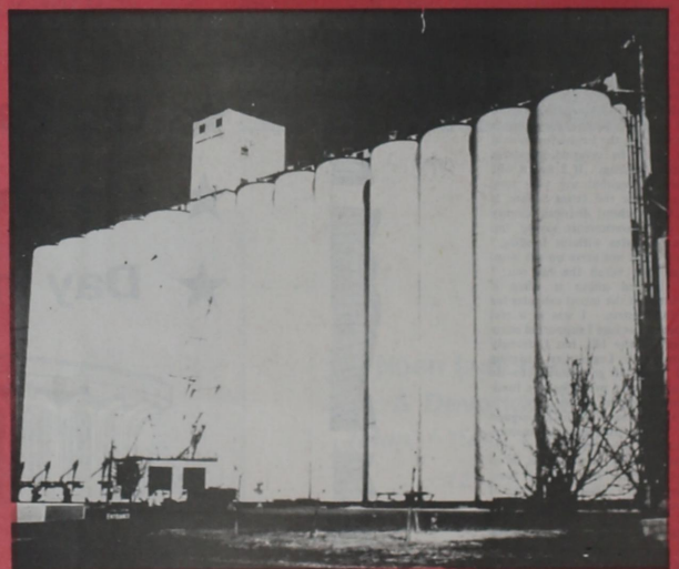
Sherley - Anderson Lazbuddie Elevator
