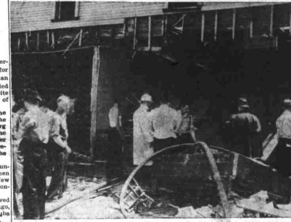
Floors buckled in a gas explosion which wrecked a frame school building in Barborton, Ohio, and some of the pupils slid to safety as if on a shoot-the-chutes. One of the "sliding" floors is shown above. Fifty-seven were injured in the explosion, several of them seriously. (Associated Press Photo.)
