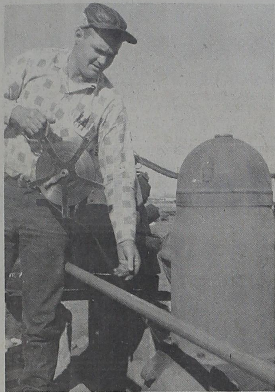
PAUL RETTMAN of the U. S. Geological Survey takes a measurement to the water table of a Parmer County irrigation well. He runs in enough steel tape down the side of the casing to reach to the level of the water. The way he determines the level is to subtract the amount of tape found to be wet when the tape is reeled back up, from the amount of tape that was rolled down into the well.
