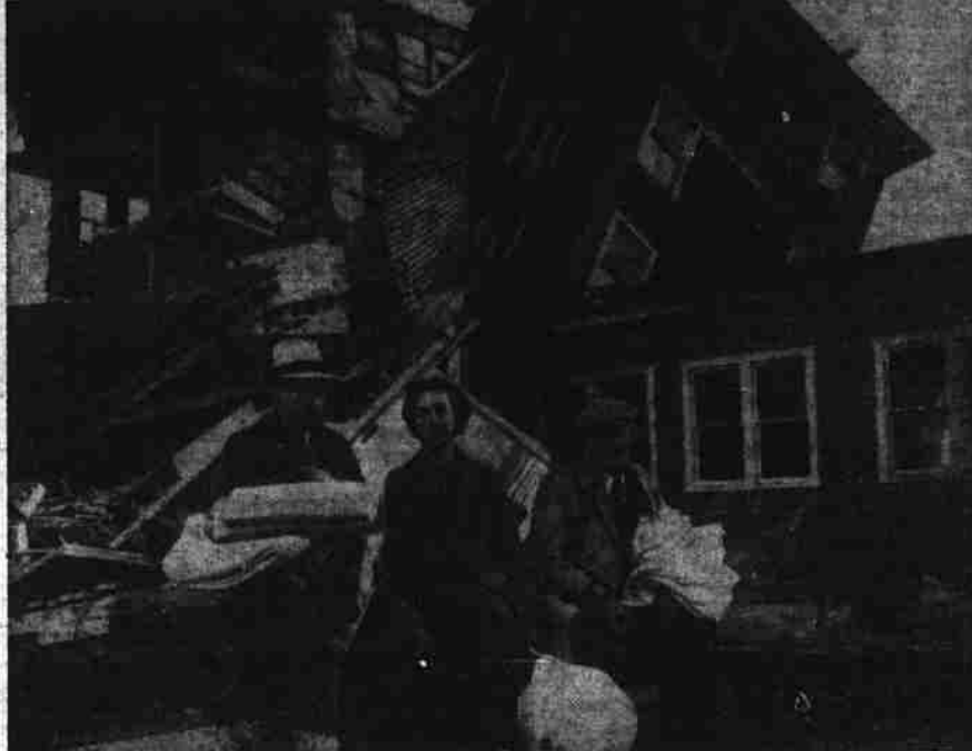
TO GET THIS aftermath of Rhode Island's hurricane scene, it was necessary to employ exceptional camera technique resulting in perfect focus of the people in the foreground as well as the damaged buildings in the background. Use of two flashbulbs plus a time exposure turned the trick.
