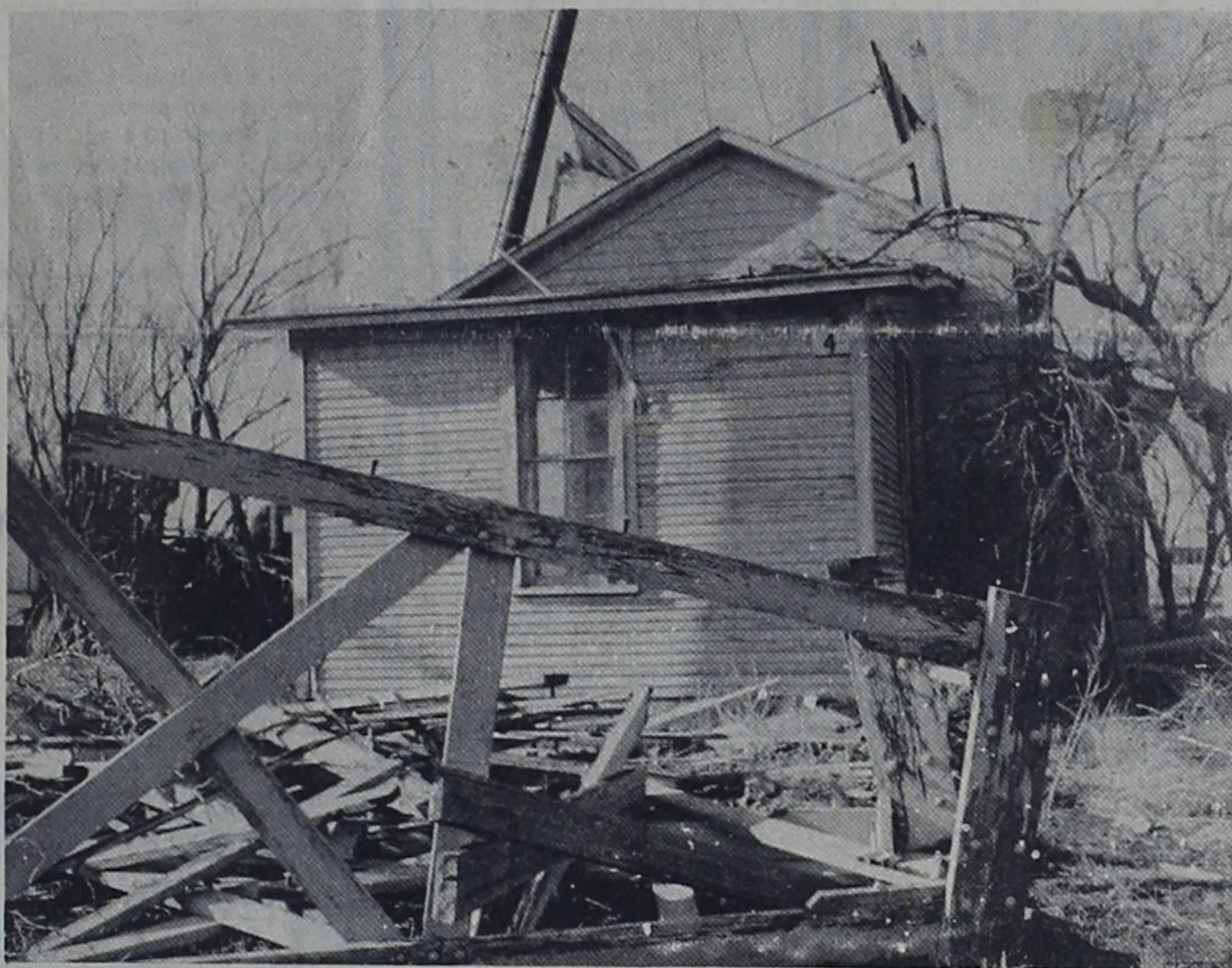
This pile of rubbish is all that remains of the water tower which once stood atop the old Santa Fe Pump House in Texico. The tower was blown from its moorings on Friday by the winds which reached tornadic fury for some three hours.
