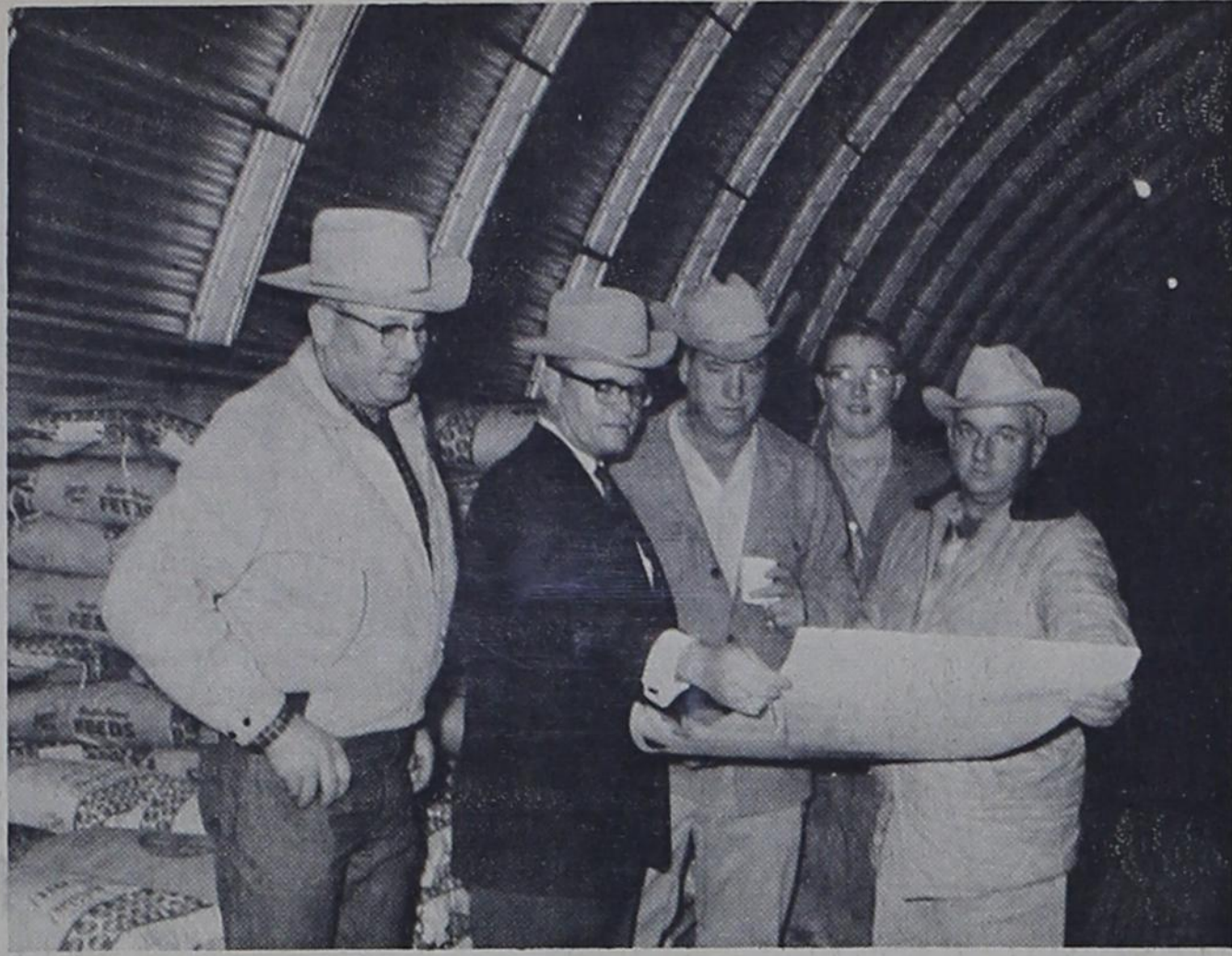
APPROVE PLANS — Gilbert Schueler, owner and operator of Interstate Distributors Farwell; James Knight, Gooch Feed Mill Representative; Bunk Phillips, Danny Schueler, and Jim McKinney, Gooch Feed Mill Representative; look over and approve plans for the new business which held open house in Farwell on Saturday. Some 282 persons registered during the day.
