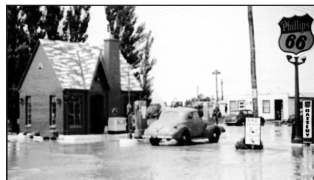
Heavy rains and flash flooding left a Phillips 66 station in Farwell flooded in this picture from the 1930s.
