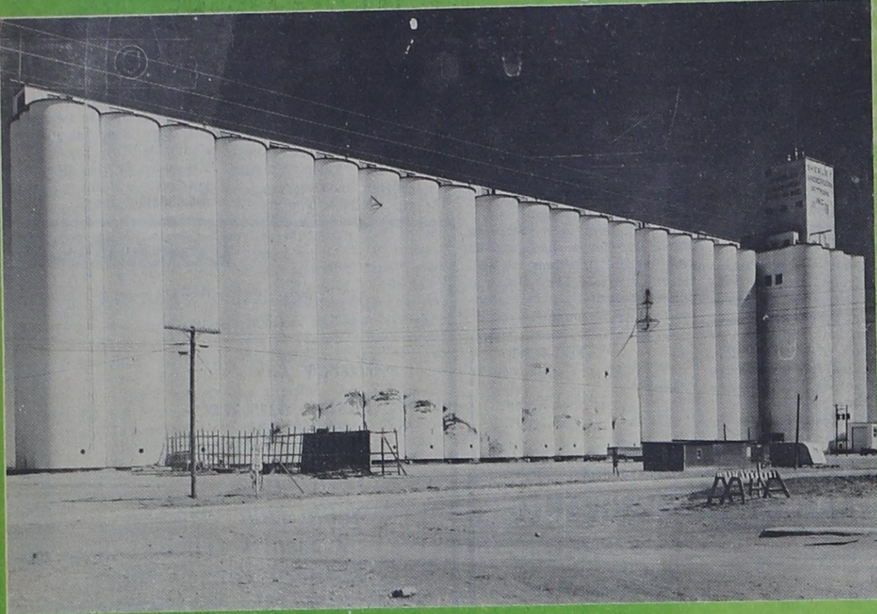
SHERLEY-ANDERSON-PITMAN, INC. - FARWELL JOHNIE WILLIAMS--FRED CHANDLER--SUSIE HAMMONDS
