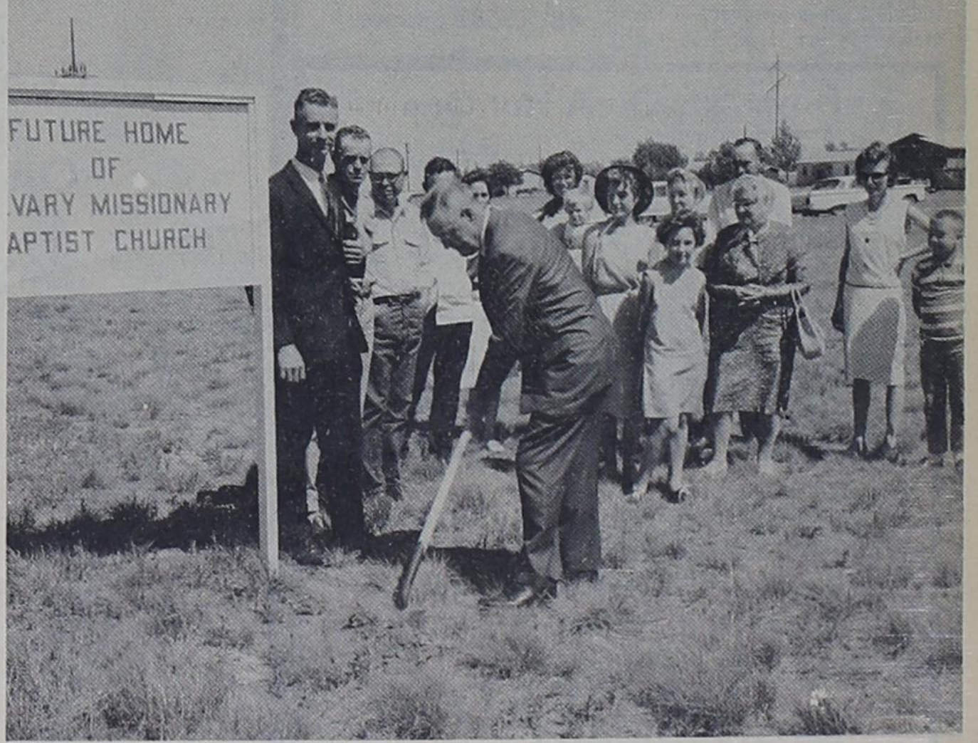
History was made Sunday when members of the Calvary Missionary Baptist Church broke ground for their new building in Farwell. Turning the first shovel of dirt is G. T. Watkins, chairman of the building committee. Near the sign is Rev. Johnny Willson, pastor. The building will be 3560 square feet in size and will be built this summer. It is brick veneer. Others on the committee are Ervin Martin and Fred Cantrell. The church has 30 members.
