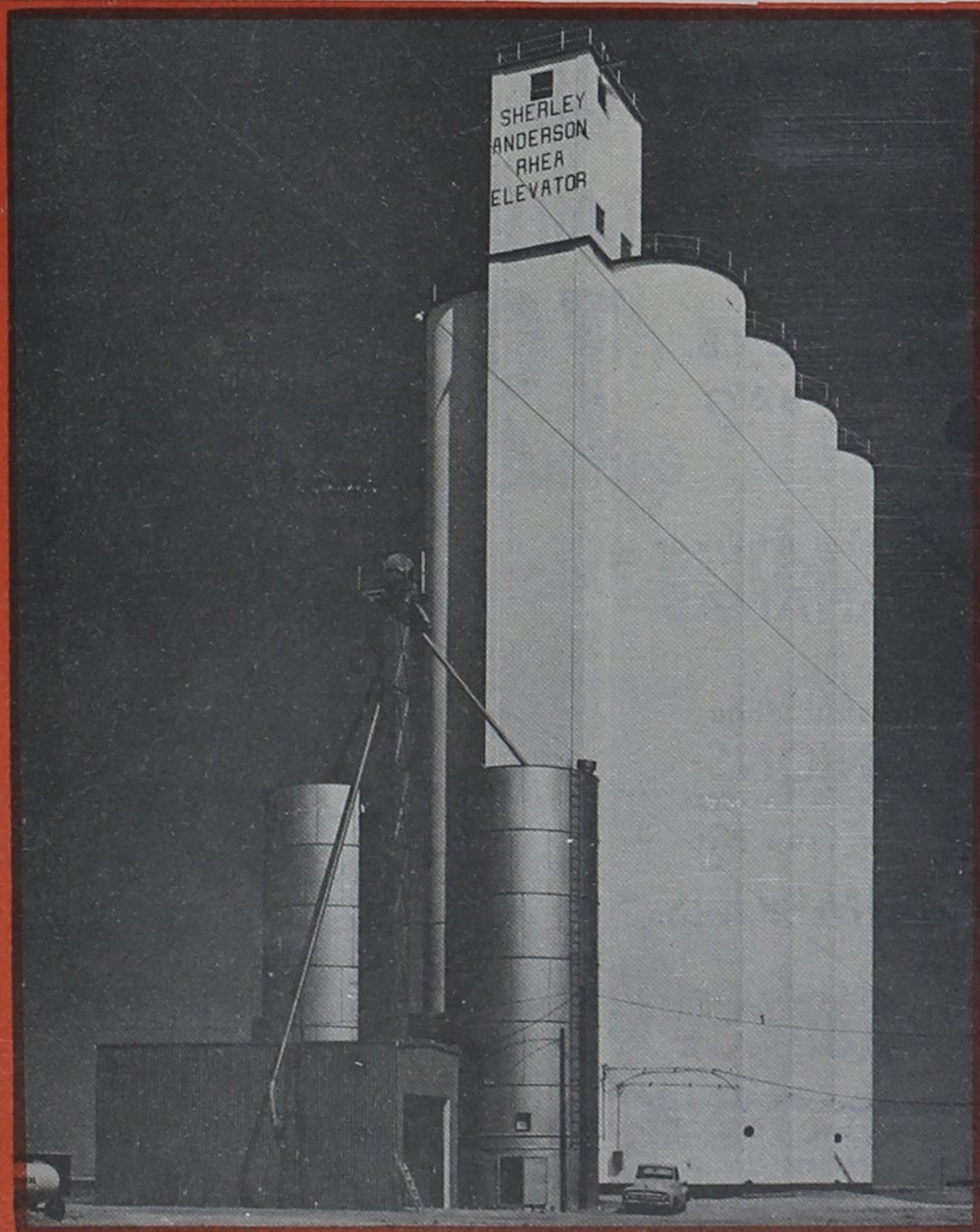
SHERLEY-ANDERSON RHEA ELEVATOR
