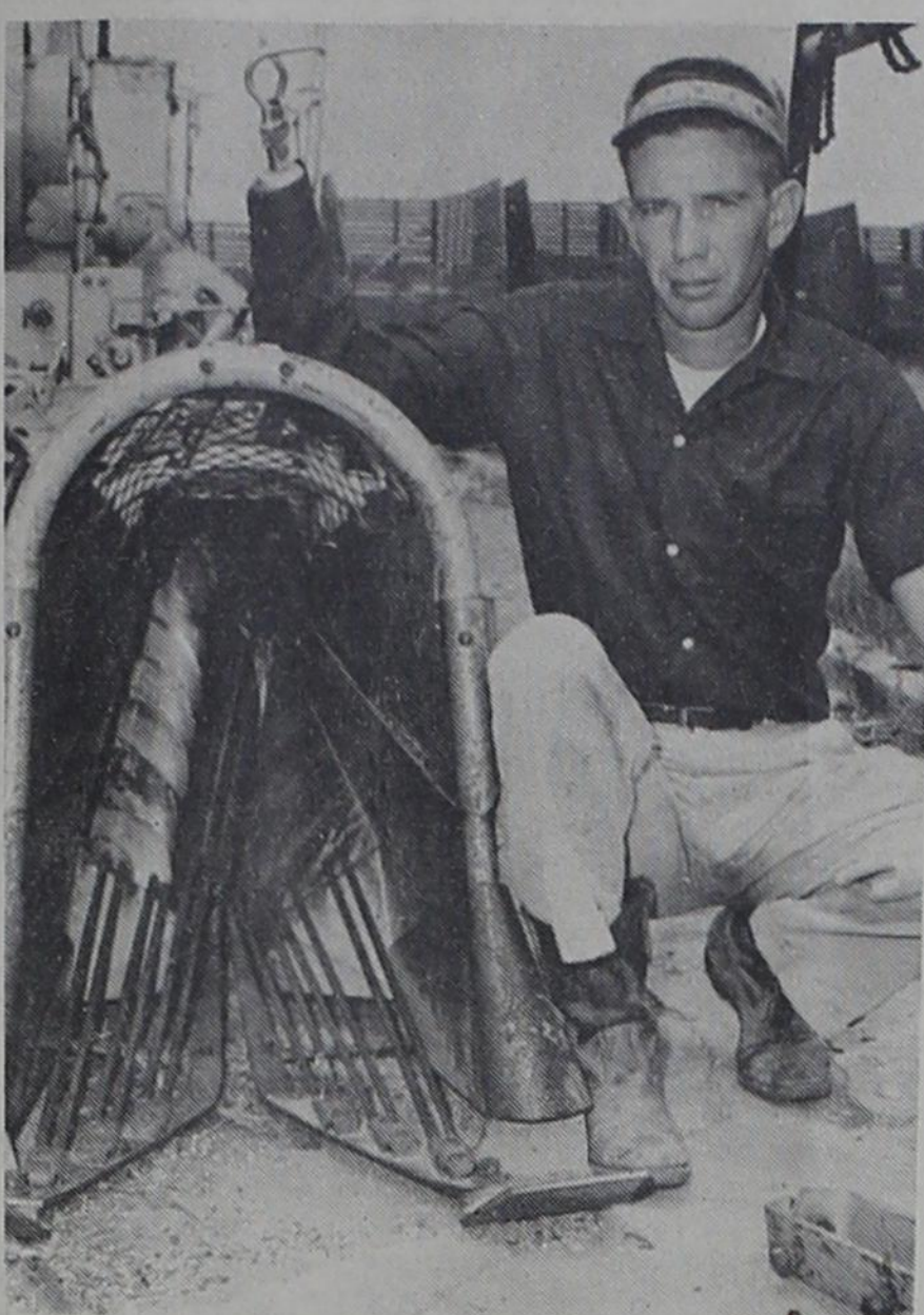
A COTTON STRIPPER AUGER isn't anything to get careless around, as Melbourn Jones will testify. Jones lost his right hand six years ago as he attempted to unstop a clogged up cotton stripper similar to this one.
