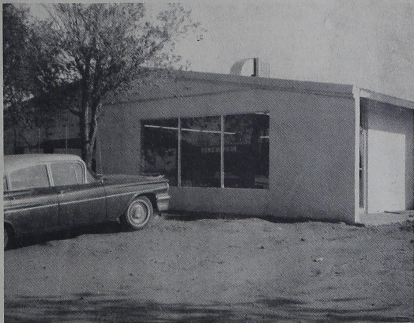
Pictured is the new concrete block building which now houses Live Longer Laundry in Farwell. The business is owned by B. V. "Shorty" Hughes. Farwell Plumbing will move into the old location.
