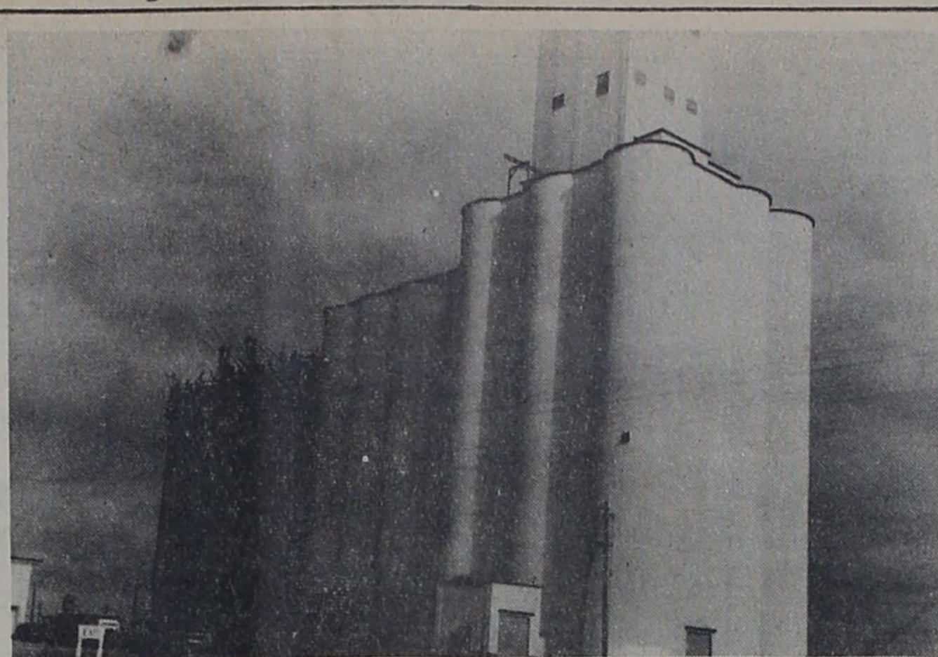
UP, UP go steel and concrete to swell Parmer County's ever increasing capacity to store grain--still the biggest crop grown here. This addition is to the Sherley-Anderson-Pitman elevator in Farwell. One sad note on this otherwise good news: a workman was killed in a fall from the construction site Sunday night.
