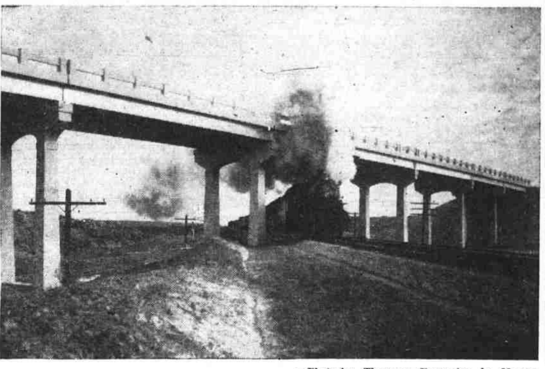
When the new overpass on rerouted highway No. 1 west is opened, there will be no more grade crossing accidents such as have claimed life and limb in the past.
