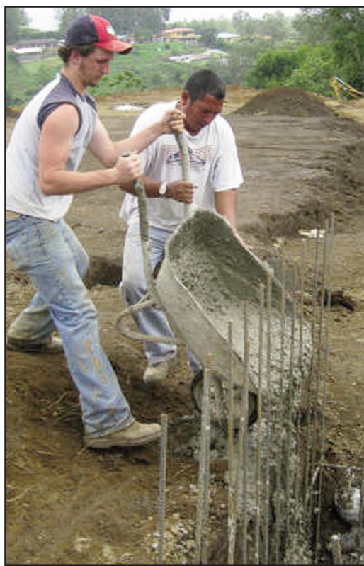
Trace Stevenson pouring concrete.
