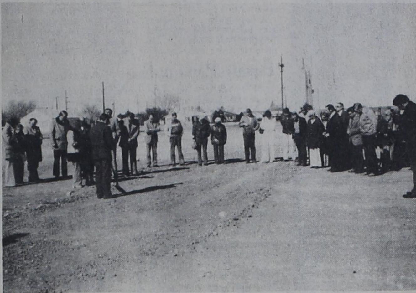
GROUND BREAKING CEREMONY - A crowd of about 45 persons stands with bowed heads as Rev. W. T. Perry gives the dedication prayer at groundbreaking ceremonies Tuesday afternoon, Jan. 27, for the 100-bed Farwell Nursing Home. The home, which has been sought by the community for several years, is being constructed at a cost of about $560,000.
